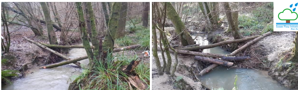
Figure 1. Leaky dam installed (left) and the same leaky dam a month later collecting debris and encouraging out of bank flow into the adjacent woodland (right).
