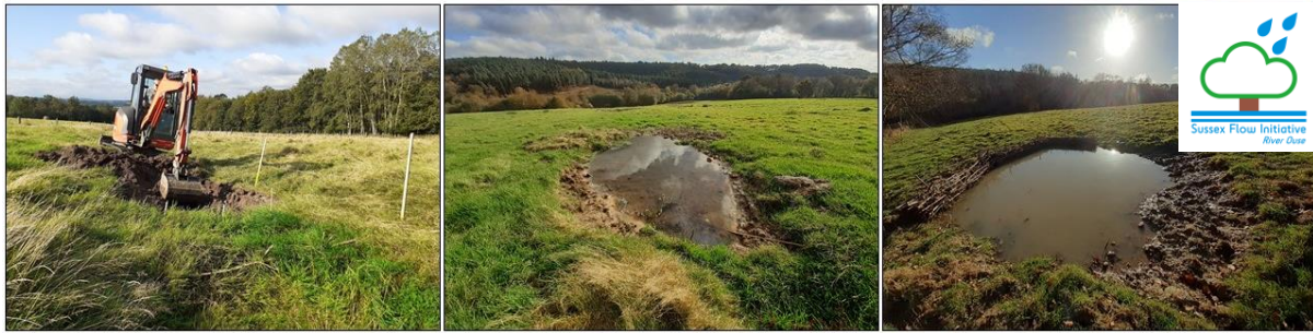
Figure 1: Breaking historic land drains and creating scrapes to store surface water [left], with (right) showing two of the thirty two completed scrapes three months later storing winter rainfall].
