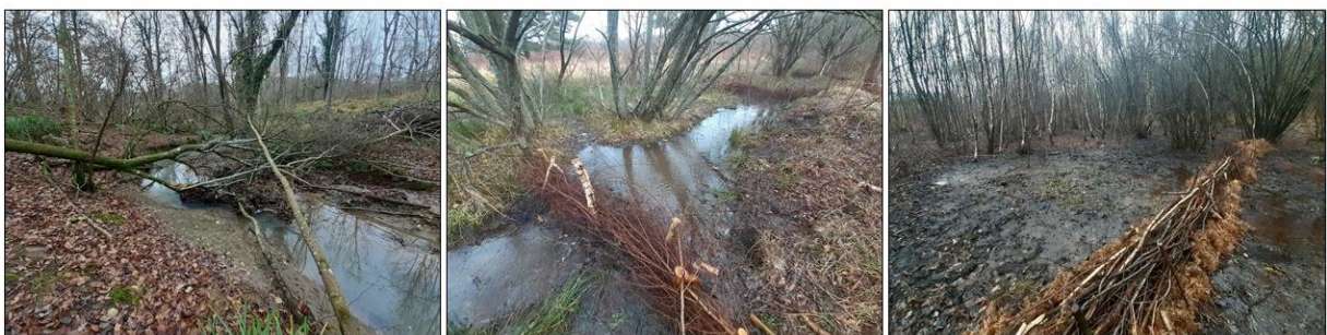
Figure 2: Leaky dams constructed this year vary from full length trees, such as this leaky dam, where the crown is restricting flow and trapping debris washing downstream (left). To smaller leaky dams constructed by local schools from brash, which are causing streams to come out of the channel and spread out (middle & right).
