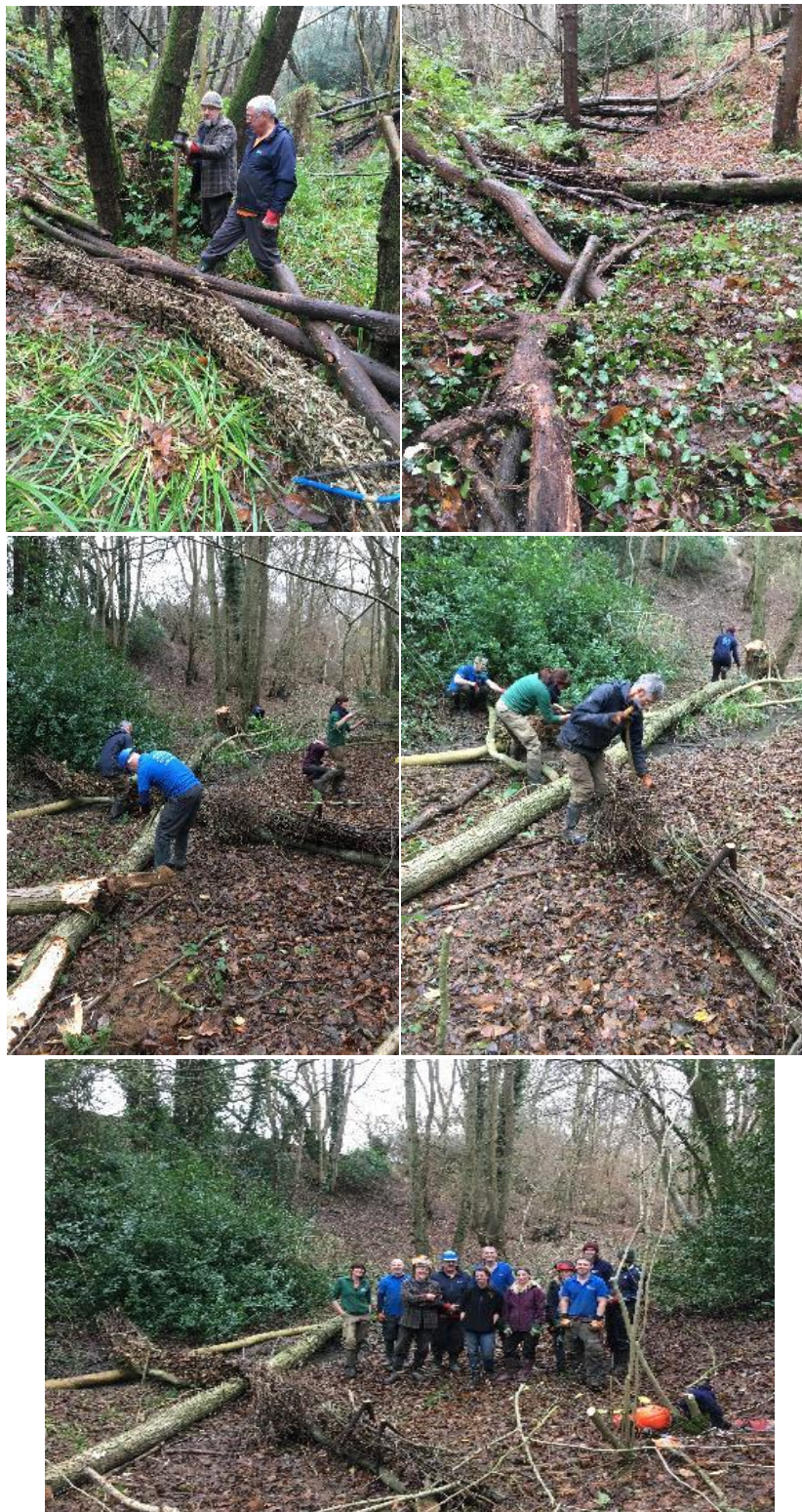
Figure 2. Volunteers installing leaky dams
