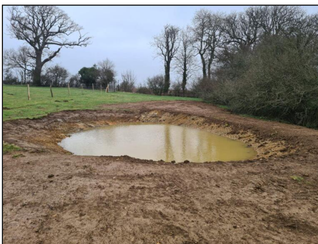
Figure 6: New pond created to capture surface water from flow path.
