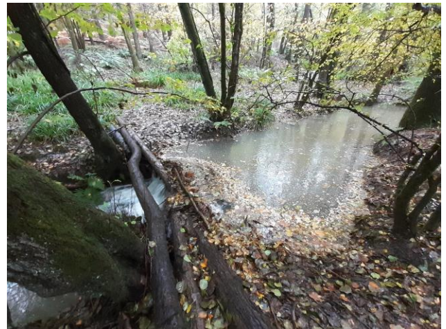
Figure 1: Leaky dam constructed to engage with high flows and engage flood waters into the wider woodland.
