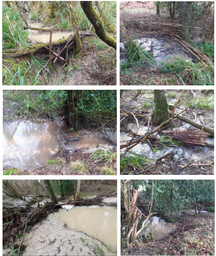
Figure 3: The variety of woody structures used to slow the flow, trapping sediment and debris.
