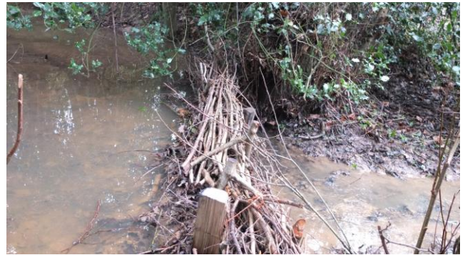
Figure 3. Leaky dam (top) and brash bundles intercepting overland flow pathway (bottom)
